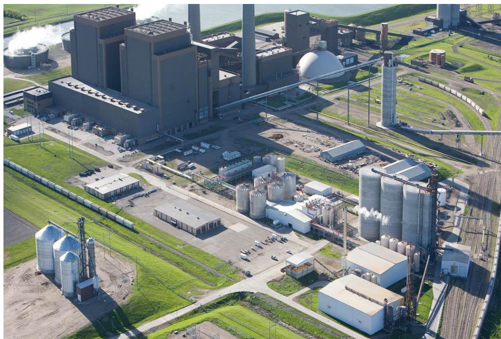
Aerial photograph of the Blue Flint Ethanol Plant with a CO 2 Capture Facility.
